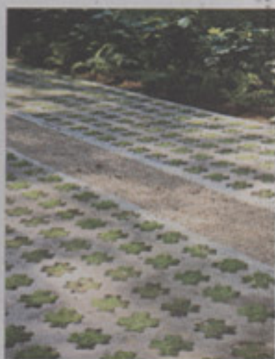
A 19th-century carriage house was gutted and turned into a studio, above. The poured-concrete driveway, right, has perforations for drainage.
